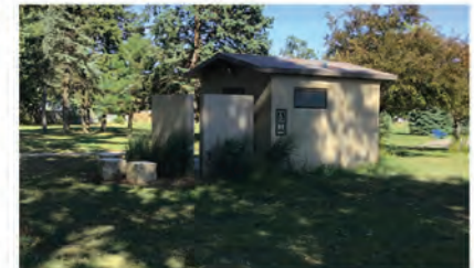
Restroom Facility PARKS CONDITION ASSESSMENT
